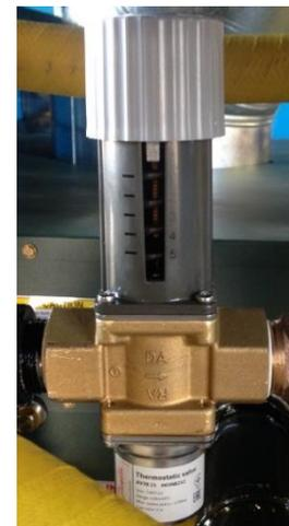
Figure 36 - Thermostatic Control Valve
