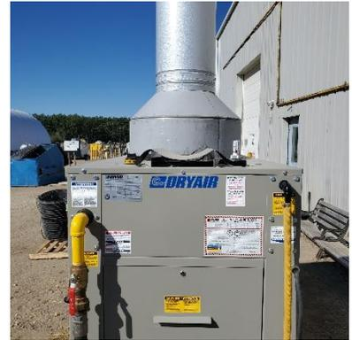
*Figure 27 - 2" Connection to Water Heater Cabinet*
