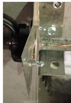
Figure 46 - Flame Roll-Out Switch
