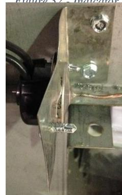
Figure 33 - Flame Roll-Out Switch
